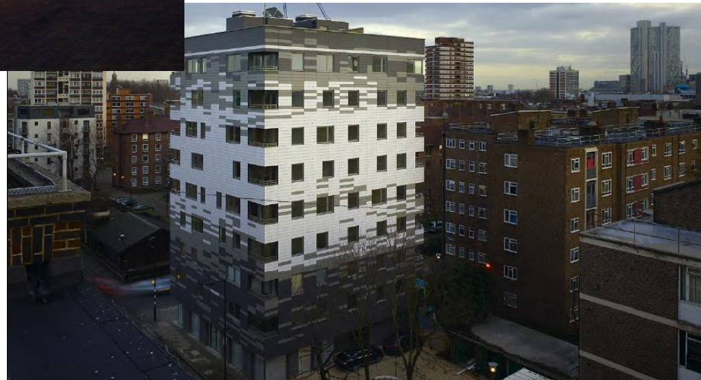
MURRAY GROVE TIMBER BUILDING- WAUGH THISTLETON ARCHITECTS – LONDON, UK
